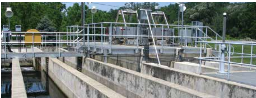
In this retrofit installation, each reactor was installed in one pass of the existing chlorine contact basin with only minor modifications to the channels. This allows the majority of the basin to be used for storage, by-pass or emergency back-up.
