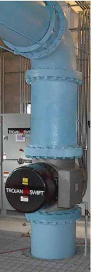
Compact footprint enables the integration of the TrojanUVSwift into restrictive pipe galleries – reducing installation costs and eliminating the need for larger buildings or additions.
